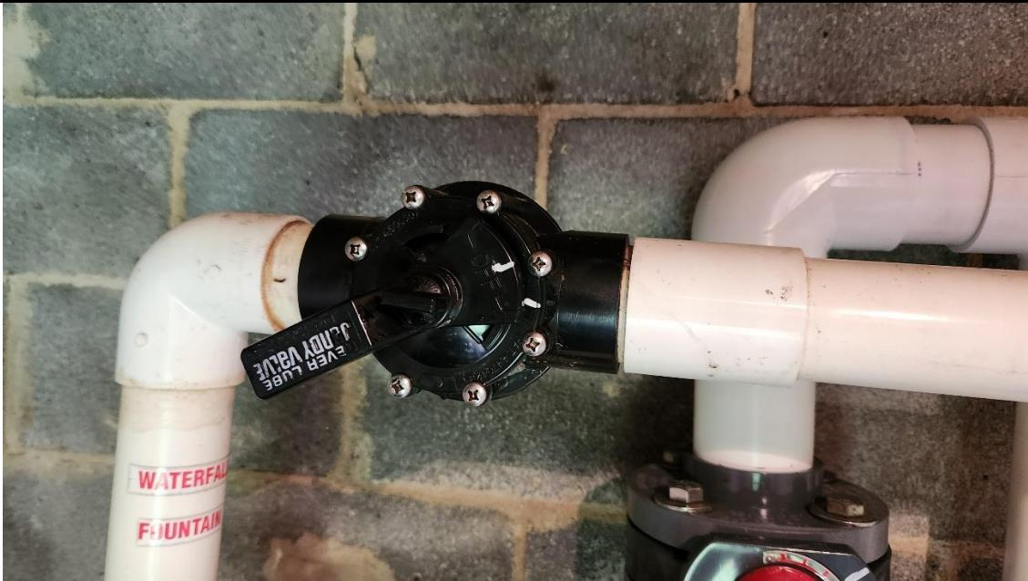
**9. Open WATERFALL LINE and re-tighten lock screw (handle should be at around 8:00 a.m.)**
