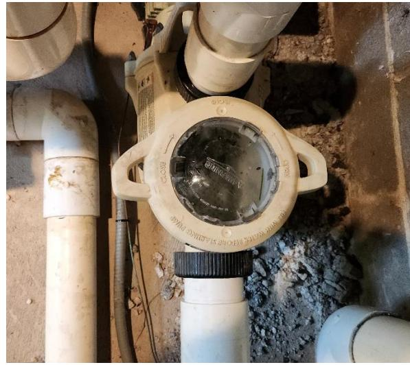
**7. Screw the strainer filter cover back on (it is indexed) in a clockwise rotation.**
