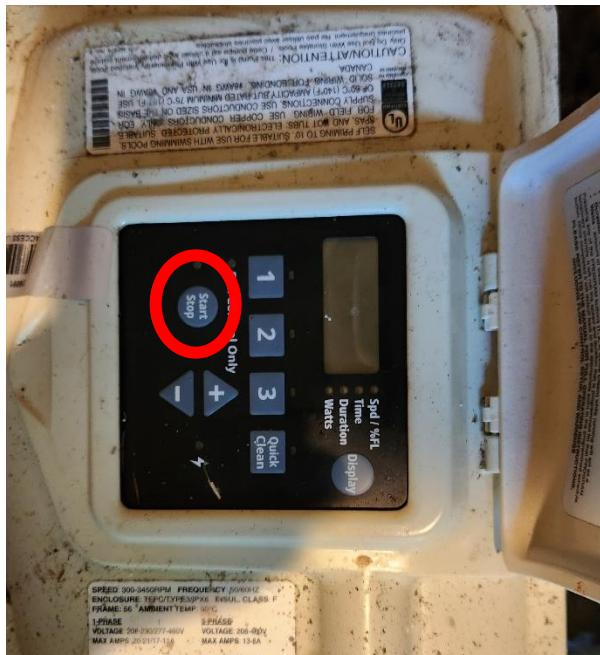
1. Open the cover to the pool pump and press the START/STOP button. Wait for pump to turn off.
