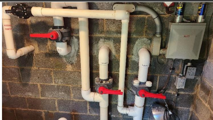
2. Close the Main Drain (MD), Skimmer line and Return line (closed position shown)
