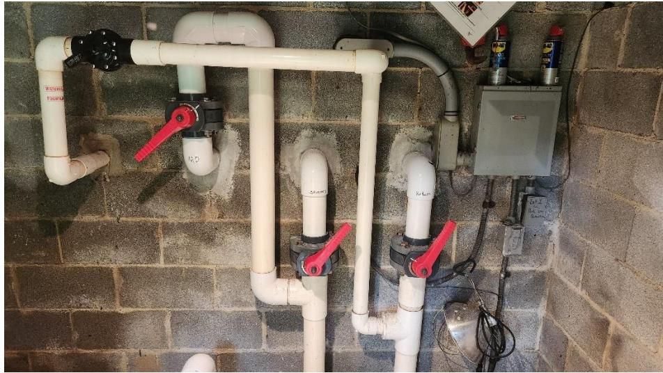
**8. Open the Main Drain (MD), Skimmer Line and Return Line to the position shown in photo**
