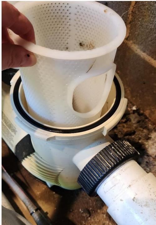
**6. Place the cleaned/rinsed strainer back in the strainer housing. Ensure the hole in the strainer matches the inlet pipe shown**
