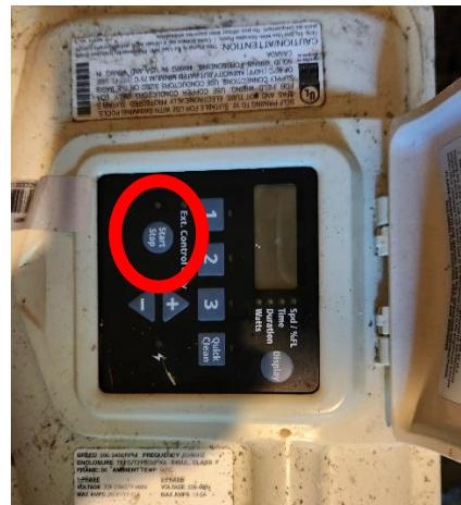
**3. Wait 30-60 seconds while water begins to flow by gravity then turn POOL PUMP to the ON position by pressing the START/STOP button. Usually there is a minor delay in the pump booting up. (Look out the door, and you will see (generally) cloudy water pumping out. Backwashing takes 2-3 minutes. Once clear water runs, turn the pump off by pressing the START/STOP button)**
