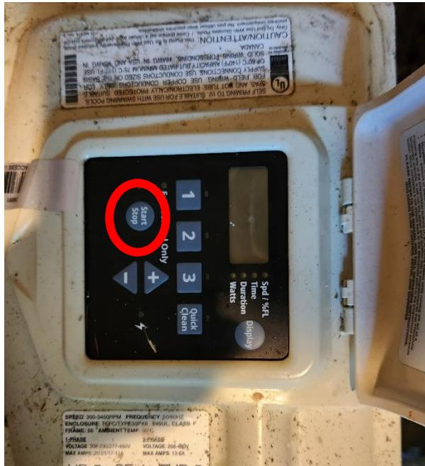
**9. Turn POOL PUMP to the ON position by pressing the START/STOP button. Usually there is a minor delay in the pump booting up. Close the cover pump cover, ensure the filter housing is not leaking.**
