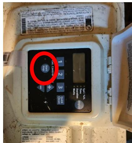
**5. Turn POOL PUMP to the ON position by pressing the START/STOP button. Usually there is a minor delay in the pump booting up.**
