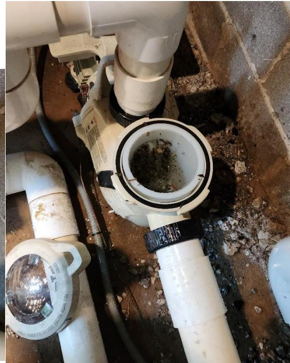
**4. Open the strainer filter housing (turning counter clockwise).**
