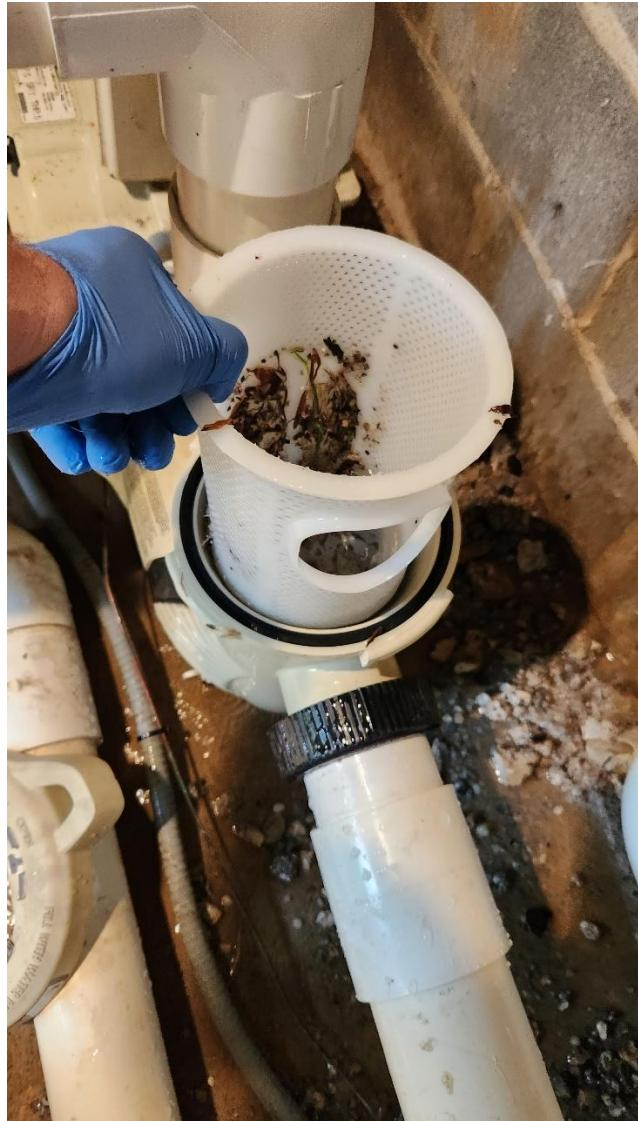
**5. Remove the interior plastic strainer bucket (there may be pool of water) and clean it out. NOTE: Pay attention to where the hole in the strainer is lined up to the pipe).**
